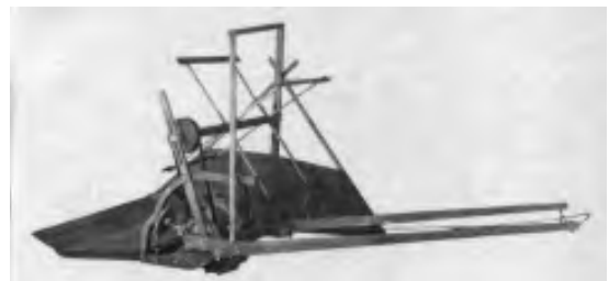
Fig.11 – Cyrus McCormick invented the reaper in 1831.
