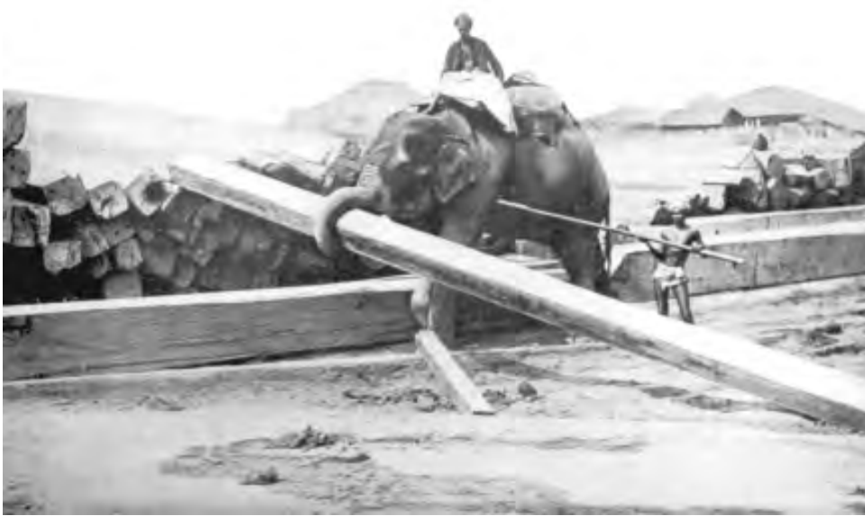
Fig.5 – Elephants piling squares of timber at a timber yard in Rangoon. In the colonial period elephants were frequently used to lift heavy timber both in the forests and at the timber yards.
