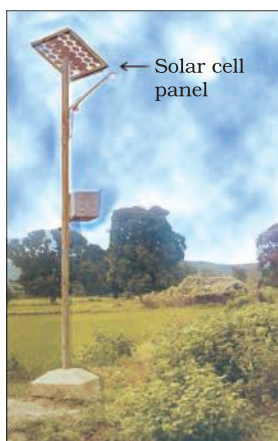
Figure 14.7 A solar cell panel
